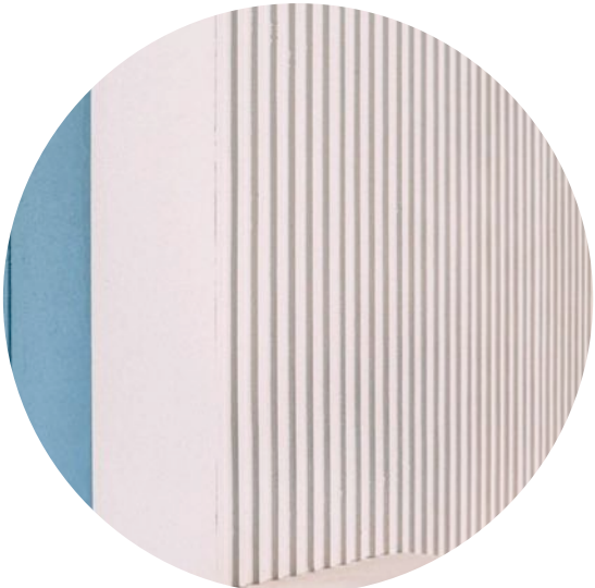
Reckli wave pattern in pre cast panels
