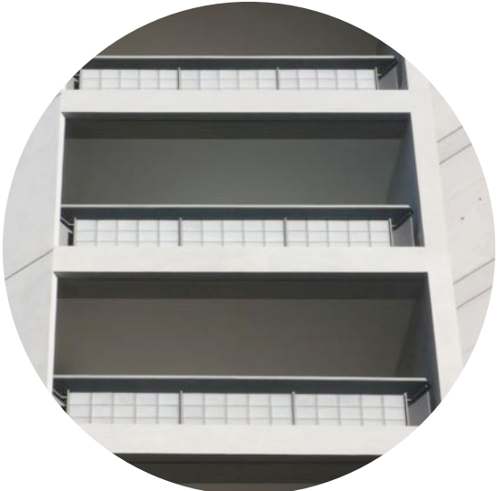
steel frame balustrade, glass block infill
